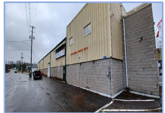
Building Envelope: MacTier Memorial Arena
