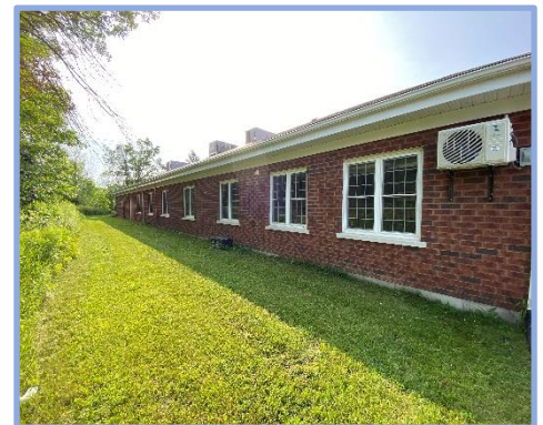
Building Envelope: Administration Building
