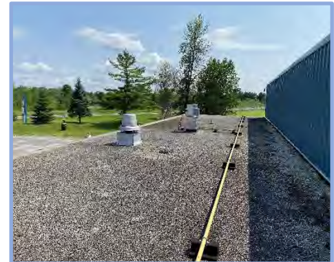
Baxter Ward Roof
