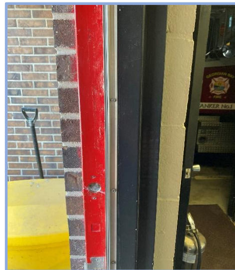
Red brick façade and concrete blocks walls
