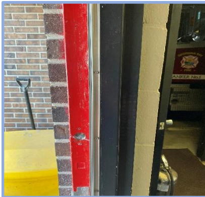
Existing block and brick walls
