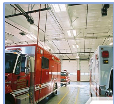
Typical metallic roof with thermal insulation
